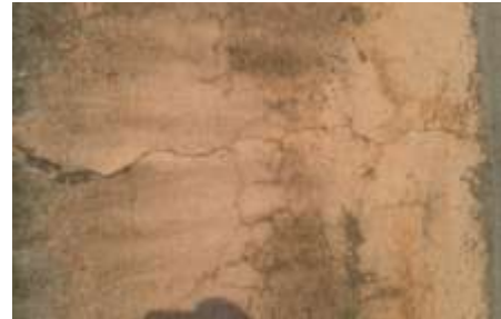
Fig.4 Plaster Crack
